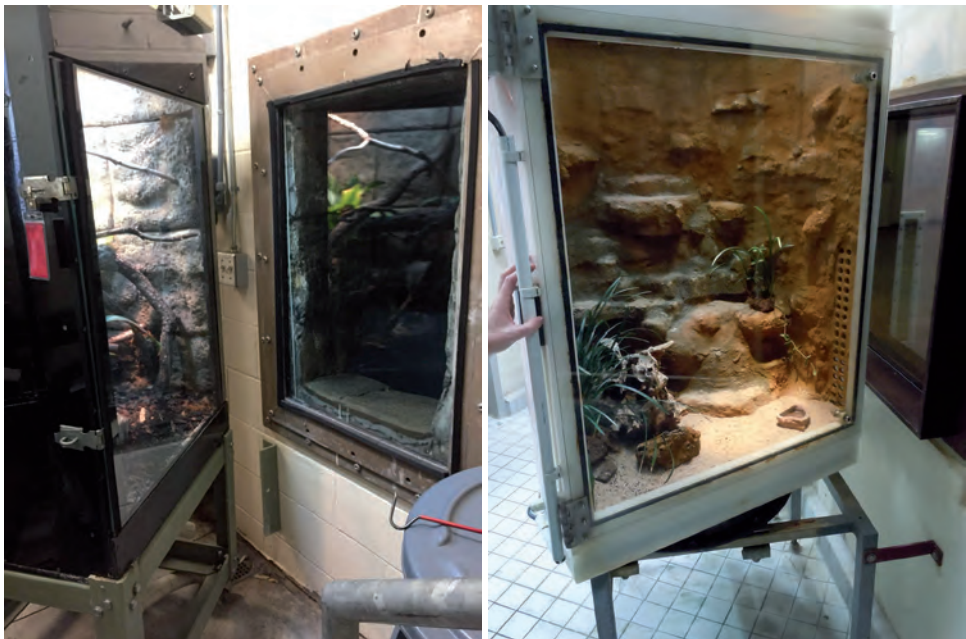
Fig 4: Examples of double-paned exhibit viewing windows for added security as viewed from behind the scenes service areas; A) exhibit on rolling casters, B) exhibit mounted on swiveling 'lazy Susan'. Fig. 4a courtesy of Emily Fyfe.
