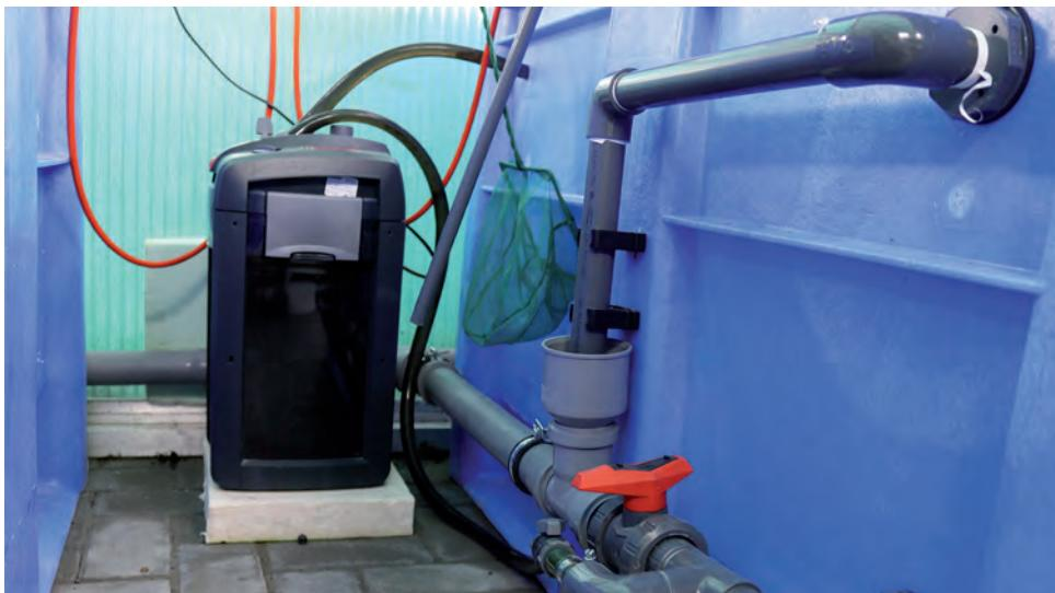
**Fig. 6:** External filter, also visible at the top right is the overflow and below it at the bottom of the tank is the drain with the possibility of shutting it off. Photo: Picture archive Aquazoo Löbbecke Museum
